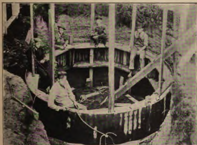
Building a silo. A project in farm mechanics in Minnesota
